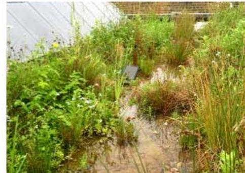
Water saturation on the green roof mimicking pond.
